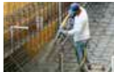
7 to 12 bar: Shotcrete applications
