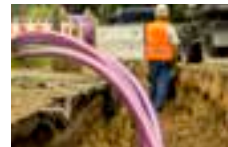
12 bar: Cable blowing and drilling
